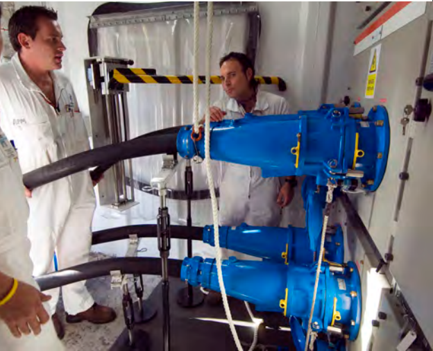
LEFT: Carnival Spirit , a Carnival ship homeported in Seattle, moors at Terminal 91. ABOVE: Enormous blue plugs provide shore power to cruise ships, so they do not need to run diesel engines to generate electricity while at berth. This helps eliminate harmful emissions from moored ships and helps preserve Seattle's air quality.
